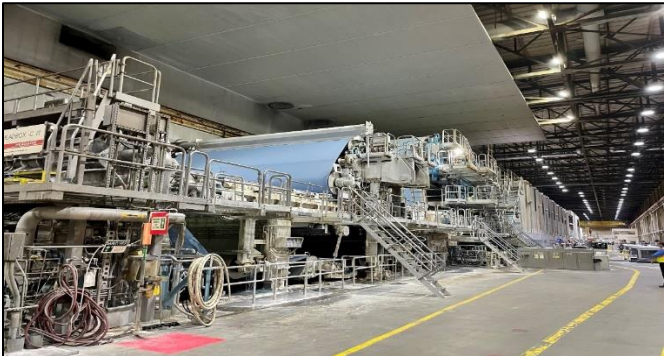
Sappi Skowhegan – Line Rebuild
